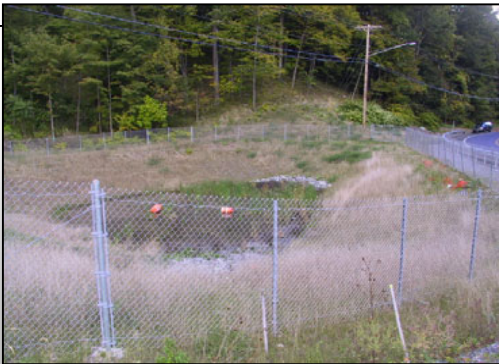
This detention basin provided a solution to the increased runoff from the NYS Route 173 project at the west end.
