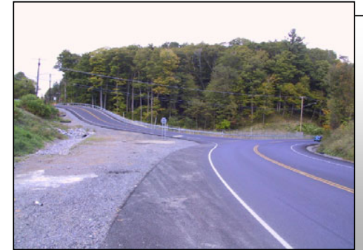
The profile was raised, the median was removed, and the horizontal and vertical alignments of the spur were improved.
