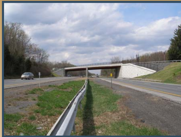
NYS ROUTE 300 OVER THE NEW YORK STATE THRUWAY (I-87)
